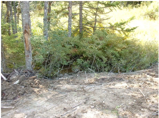
The upgradient area of this wetland was not properly stabilized and maintained, causing large amounts of sediment to deposit in the wetland. The cost to retrofit this stormwater structure will be more costly than if the original specified construction and maintenance plan had been followed.
