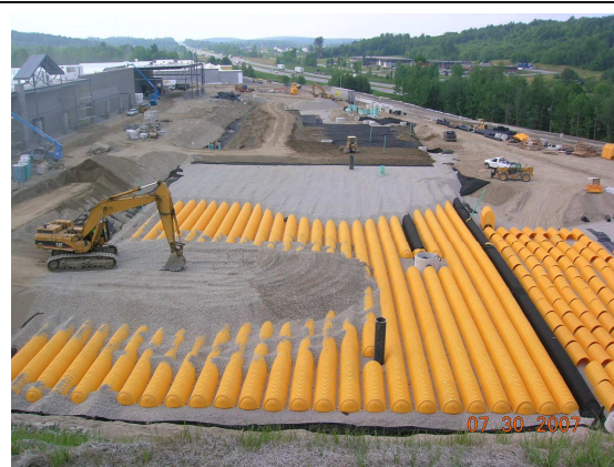
Subsurface detention and infiltration galleries under a parking lot save space. With visible and adequate pretreatment and frequent maintenance, they can work well and will help recharge groundwater. Without pretreatment and maintenance, they quickly fill with sediment and may fail.
